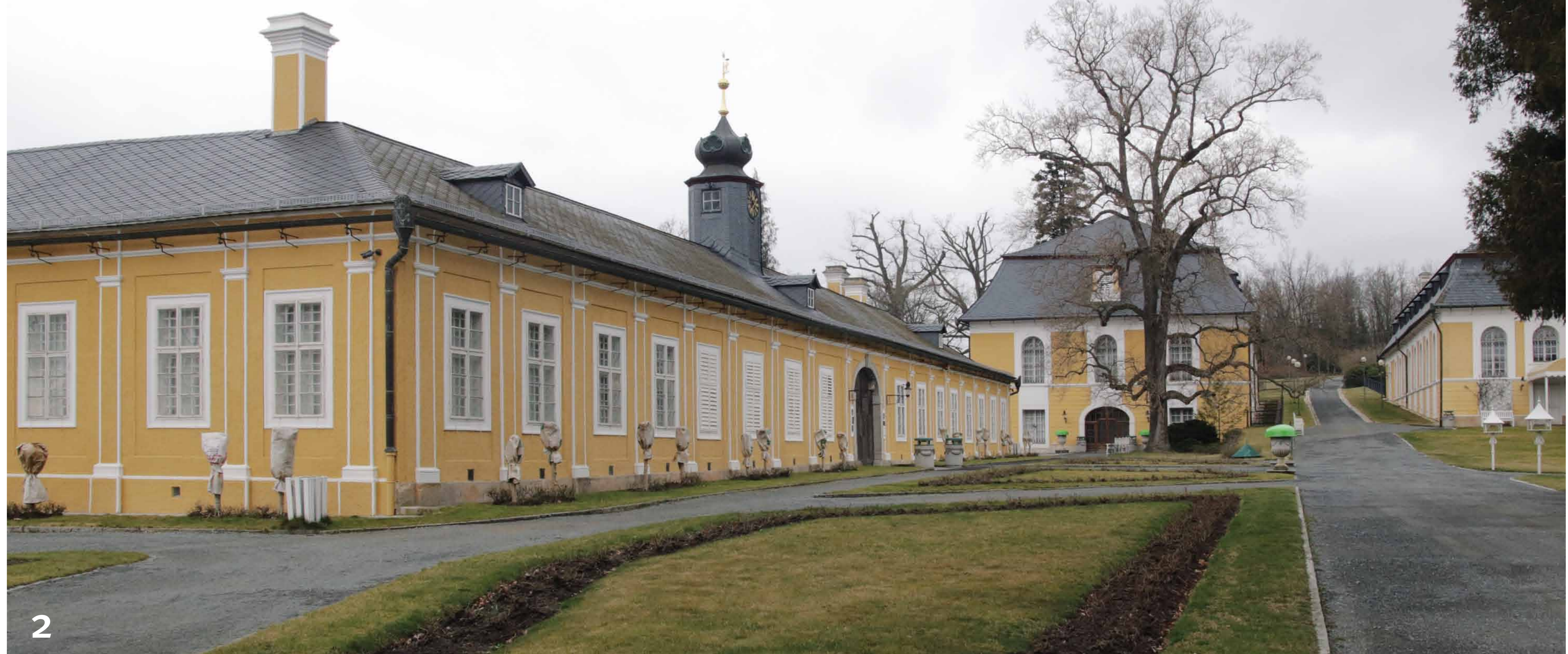
2 The theatre is located in the front wing of the hunting lodge
